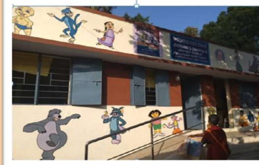
AWC with RAMP facility
